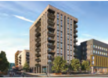
Rockcliffe Square Plumstead lqhomes.com/rockcliffesquare
