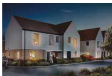
The Arbour, Chelmsford lqhomes.com/beaulieuarbour
